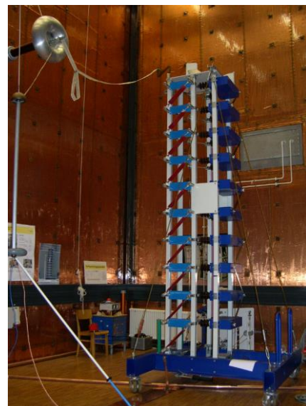
Figure 1. 1 MV Marx impulse generator [11].
