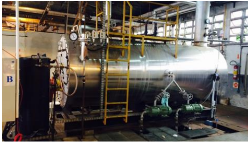
Figure 2. Diesel boiler at the power plant of Sao Tiago Polydoro Ernani Hospital.
