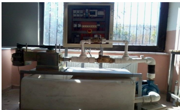
Figure 6. Closed loop MHPP general appearance of the prototype.
