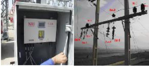
Figure 2. Test site, the sample insulators and monitoring equipment.
