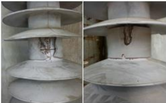
Figure 8. Defective sealing increase high rate of moisture ingress.
