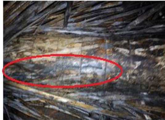
Figure 10. Mechanical cracks in varistor elements.
